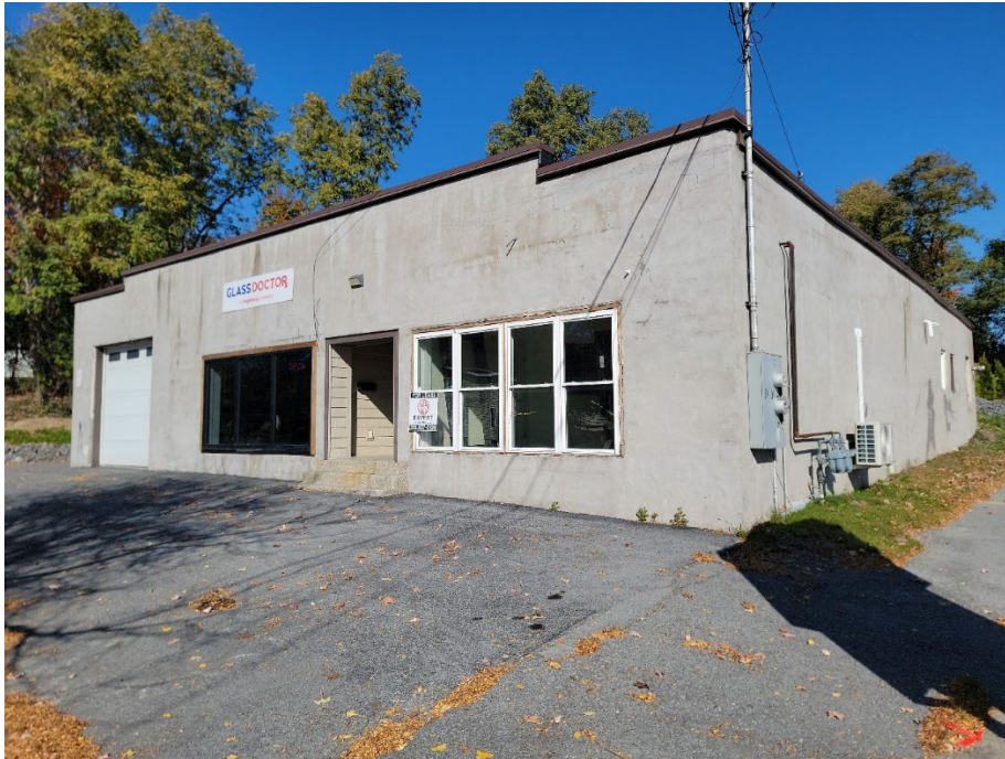
Above: Picture of the store front from the front, looking north.
