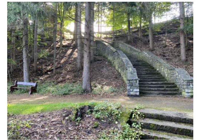
The historic stairs are an iconic fixture in Thompson Park
