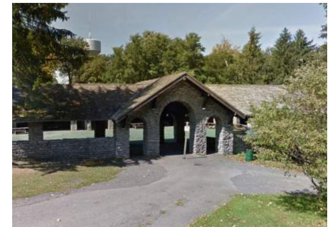
The Horse Shed is renovated and repurposed as a Picnic Pavilion
