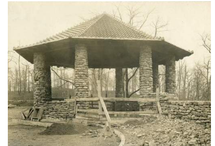
Historic photograph of Pinnacle under construction
