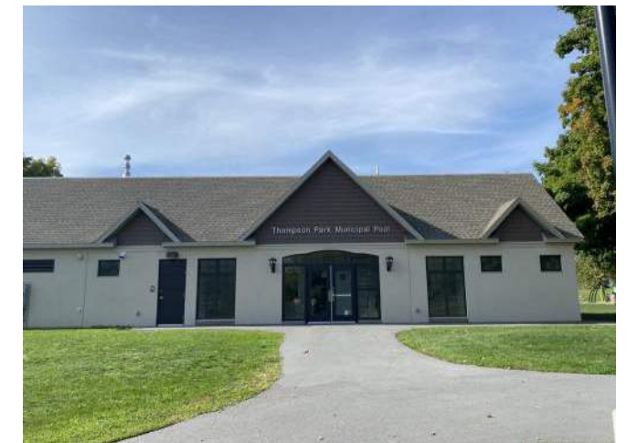
View of the existing Bath house
