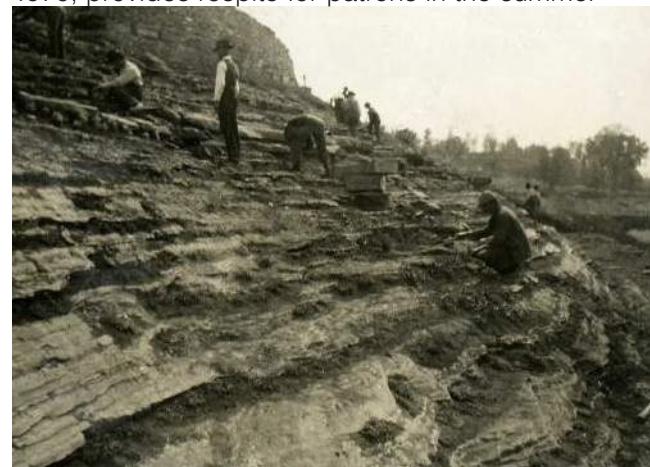
North Outlook Cliff Garden is partially constructed
