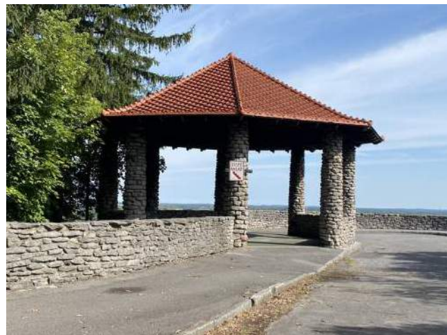
The Pinnacle Overlook road pavement and curb need alignment.
