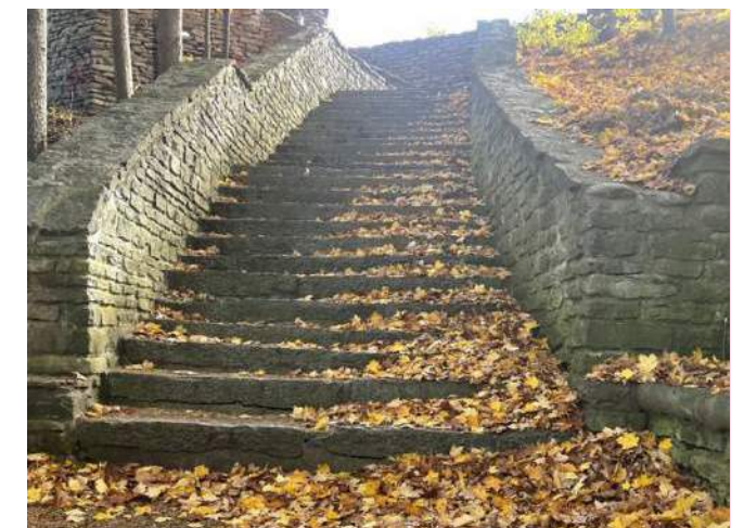
Stairs are generally in good condition
