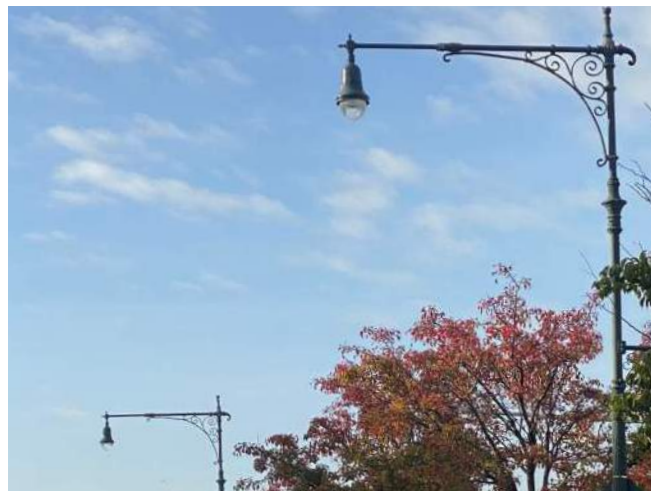
Type M Roadway Luminaire
