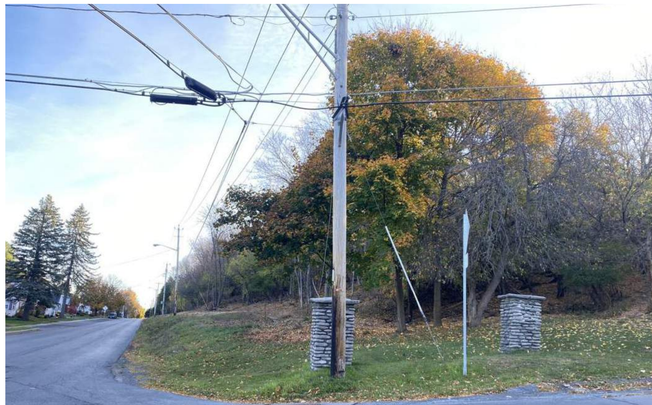
Existing conditions at the corner of Gotham Street and Thompson Boulevard, Fall 2022
