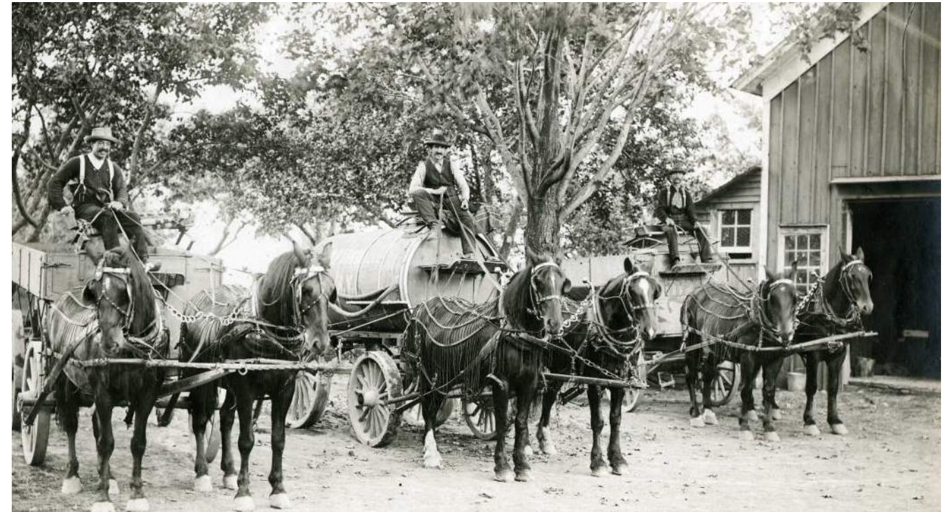
Construction team, 1902. Image courtesy of the National Park Service, Frederick Law Olmsted National Historic Site
