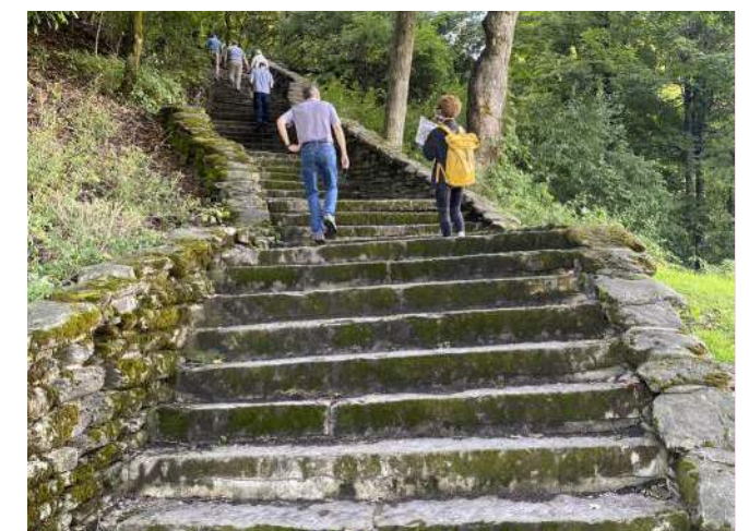
Existing stone stairs with monolithic stone treads
