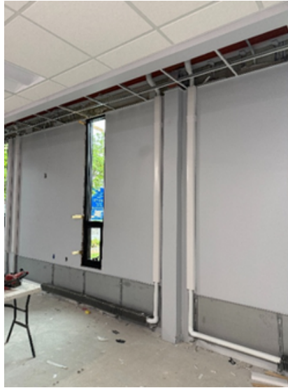
Wall & Utility Improvements
