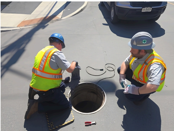
CSO Maintenance and Inspection
