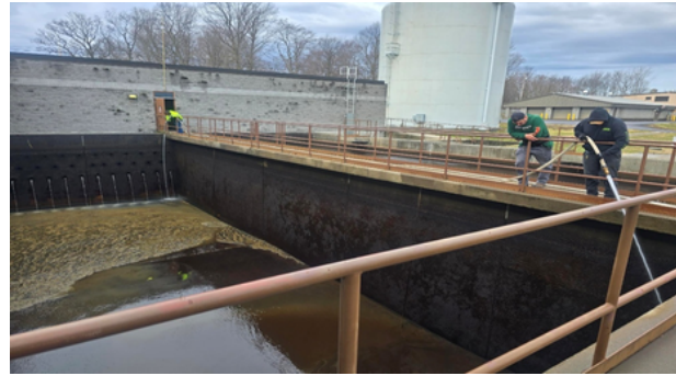
Coagulation and sedimentation tank maintenance and cleaning (Contact Tank)
