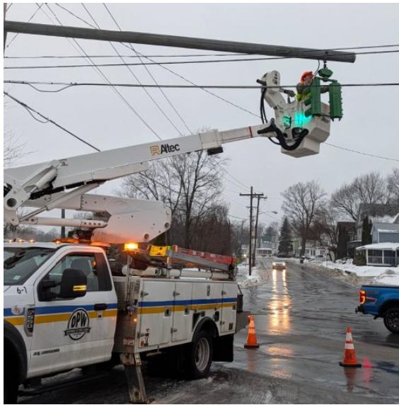
Signal Maintenance is an important aspect of winter work. Fluctuating temperatures can affect signals and their functions. Windy conditions can also cause signals to be dismantled or unaligned.
