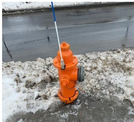
Staff have continued to repair hydrants and remove snow from 890 hydrants around the city. Pictured below is a Kennedy Hydrant damaged that had the collision ring replaced.
