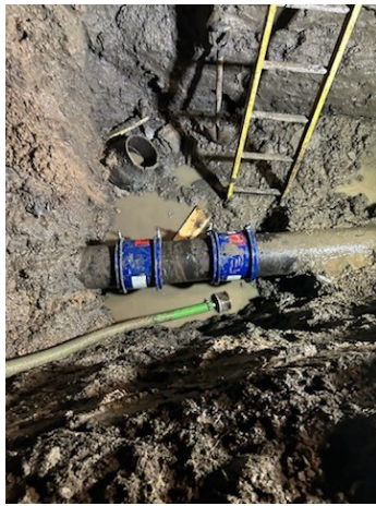
On December 6 and 11, staff repaired the 10-inch main, once at Starbuck and Seward and once at 725 Starbuck.
