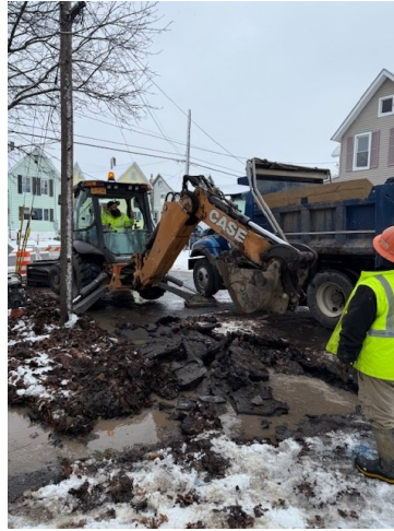
On December 6 and 11, staff repaired the 10-inch main, once at Starbuck and Seward and once at 725 Starbuck.
