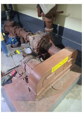
Older equipment occasionally needs extra attention. Operations and maintenance staff at the Pollution Control Facility recently responded to an issue with Primary Digester #1 recirculation pump, which had gone out of service. The team identified a blown fuse and a worn drive belt, completed the necessary repairs, and returned to pump to full operation. Proper digester mixing is essential to ensure organic matter breaks down to levels that meet DEC and EPA regulatory requirements.
