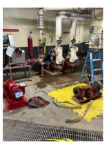
Operators at the Wastewater Treatment Plant (WWTP) replaced the hot water pumps for Primary Digester #2's heat exchanger. The digesters play a crucial role in stabilizing biosolids, making them suitable for beneficial reuse. Experienced staff used this maintenance project as an excellent training opportunity for junior team members.
