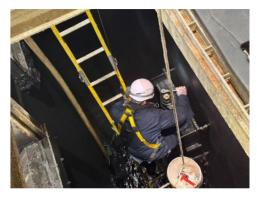
WWTP staff replaced the bearing for Trickling Filter Gate 2 and removed the shaft due to excessive wear, which will be replaced with a new stainless-steel shaft. Gate 2 enables the alternating of trickling filters between lead and lag positions. Alternating the filters enhances biological water treatment by maintaining a more even distribution of biological growth across the filters.
