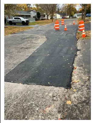
DPW has paved the area surrounding the new catch basins, and construction for this project is complete.
