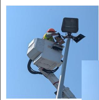
DPW electricians have been out replacing old inefficient parking lot lights with new LED. These new LED's are not only better on electric usage, they also provide more lighting coverage.
