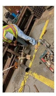
Leak studies are being performed by staff to invenstigate for main breaks or leaks on in the distribution system. The discontinued service to Nice and Easy on outer Bradley St. has been isolated and the meter removed after department staff identified the service to be leaking.
