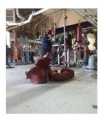
New discs were replaced on secondary digester transfer pump.
