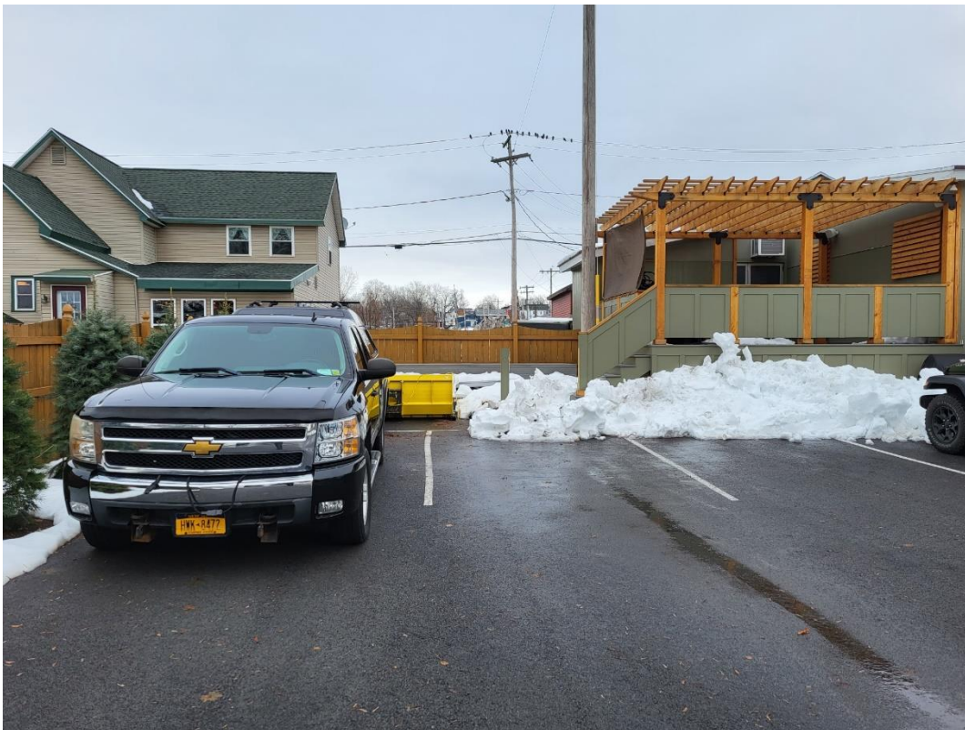
Below: The newly constructed deck and the area where the applicant proposes planter boxes.
