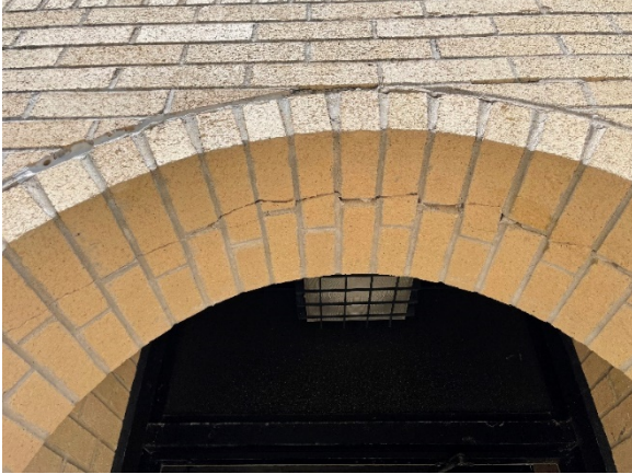
Crack in Brick Veneer
