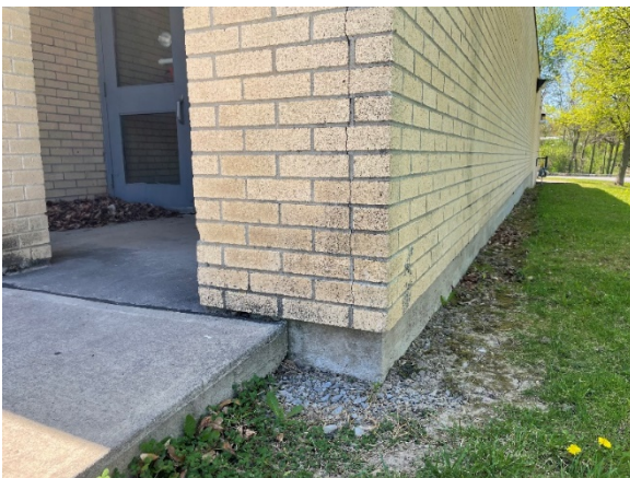
Vertical Crack in Brick Veneer
