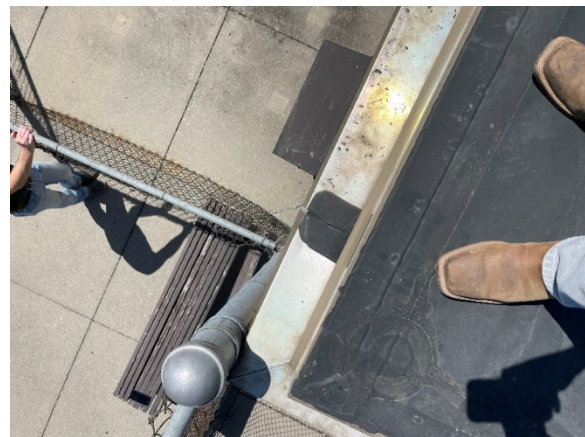
Split Rubber Flashing on Edge (Typical)
