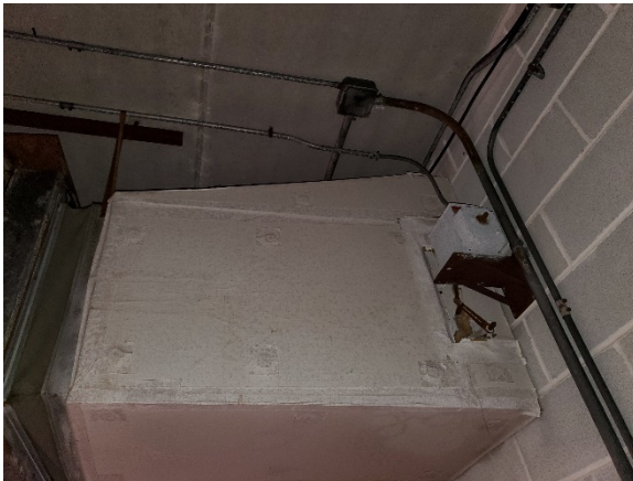
Filter Room Ventilation Unit
