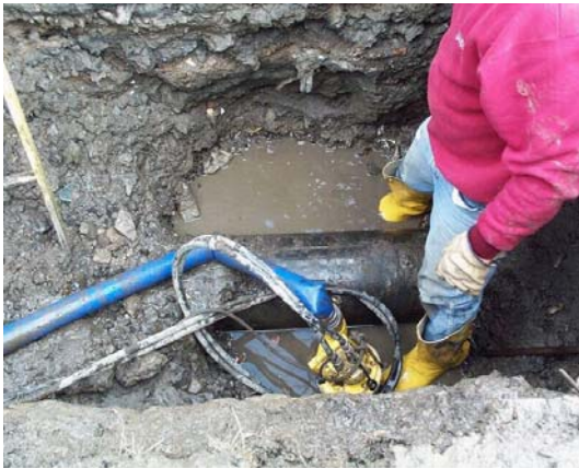
Successful location of leak and shut down of main.
