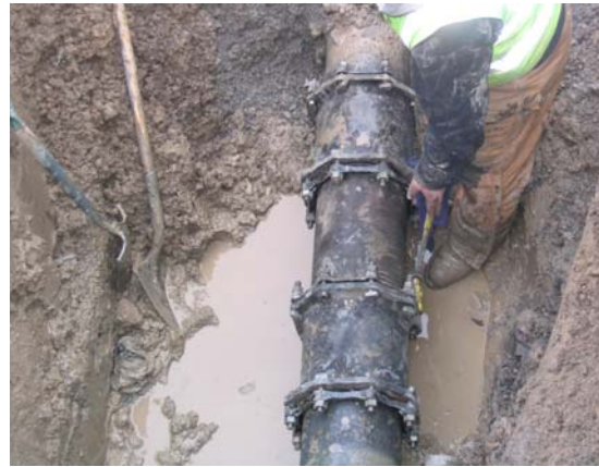
Tightening the last bolts on the repair sleeves.
